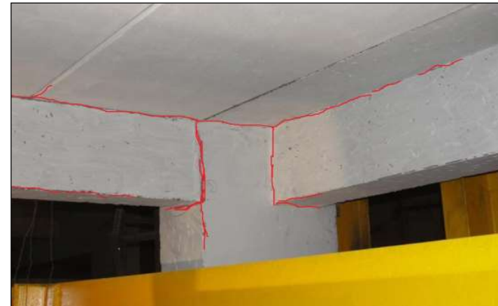
Wide cracks at beam-column junction- inner face
