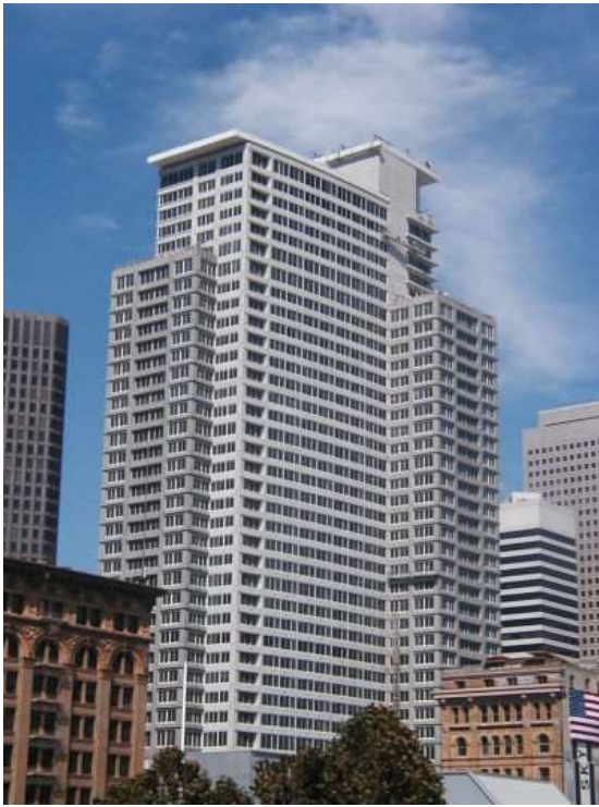
The Paramount Tower - 39 story moment frame San Francisco, California
