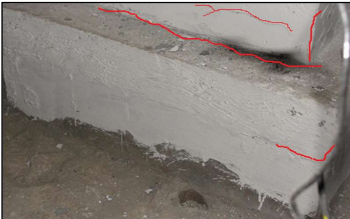
Minor horizontal cracks at junction of pedestal and column
