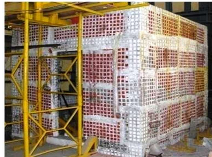
Application of Plastic Cement Bag Mesh™
