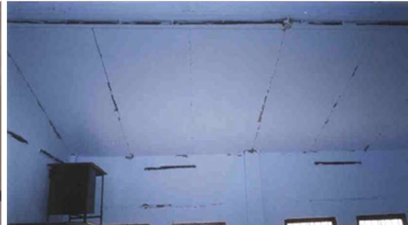
Type B – Slipping of roof planks
