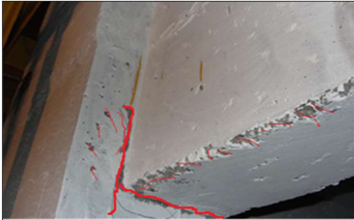
Crack at beam-column junction- outer face
