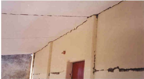
Type A – Major damage to structure
