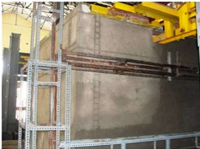
Plastering and Curing
